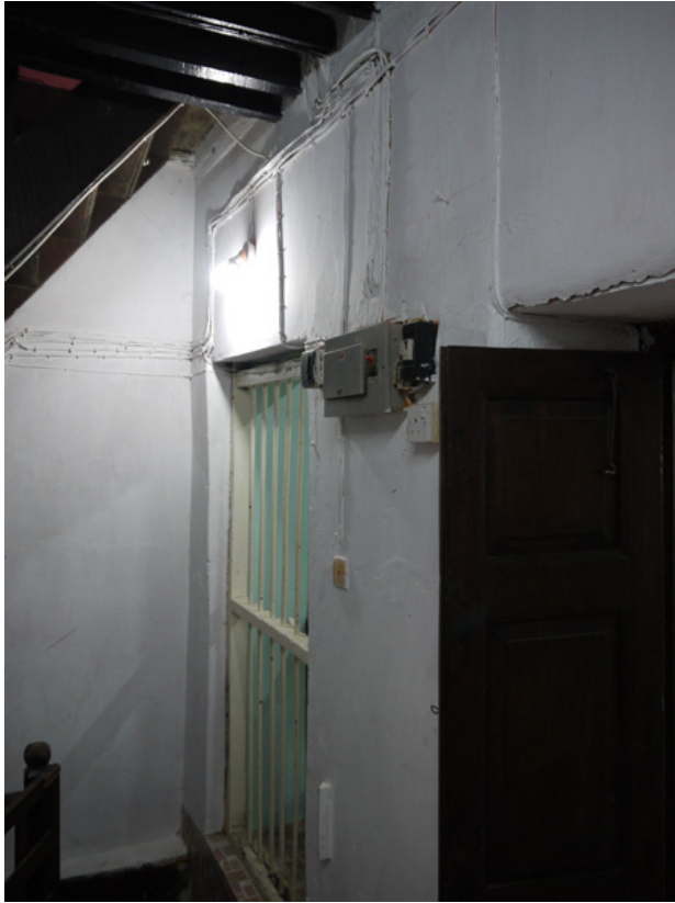
Figure 3. Interior view of a house in Stone Town, Zanzibar featuring LED light fixture and improvised electrical wiring connected to PV collection cells. Image by author, 2011.
